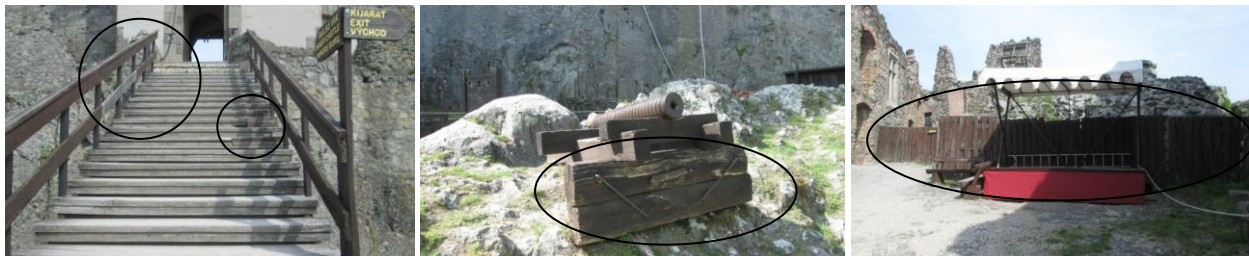
Photo 15 some parts of the monument need corrective maintenance works (especially for wooden structure)
