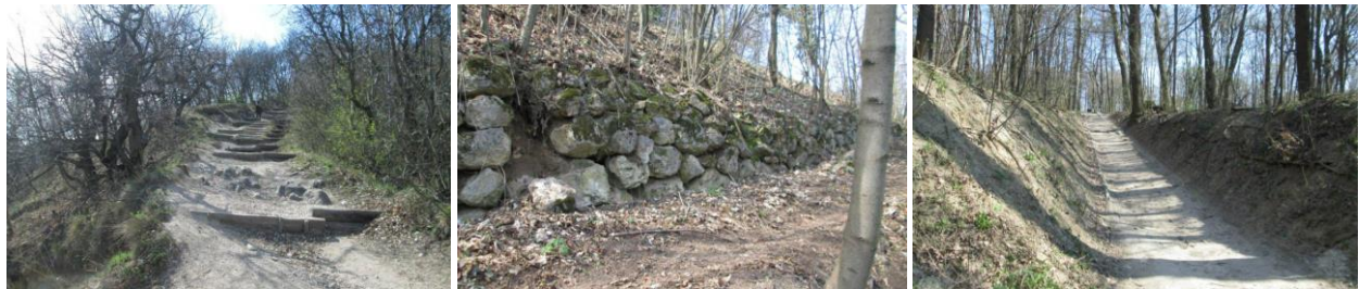
Photo 5 some part of normafa trail routes need preventive and corrective maintenance works to protect soil erosion.
