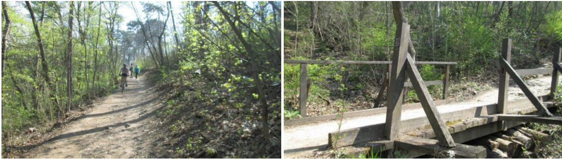
Photo 12 the same route for walking user's and cyclist had created conflicts among park user as well as broken hand rails wooden bridge causes dangerous to walkers
