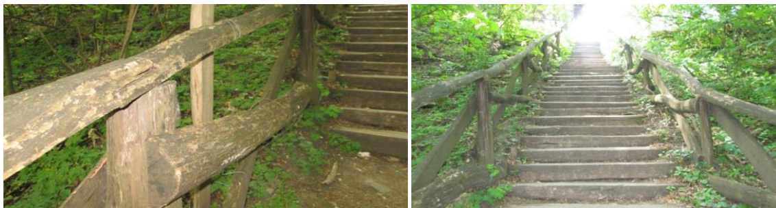
Photo 18 wooden hand rails being found requires corrective maintenance due look dull and some part had broken
