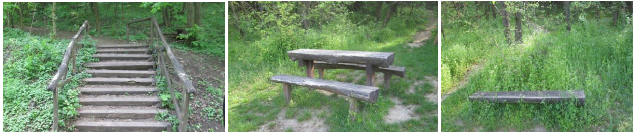
Photo 17 some of the elements need corrective maintenance due to going to dull and decaying. Some of them look like abundant.
