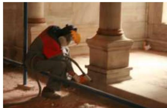
Figure 6: Interior sandblasting (Güneş, 2011).
