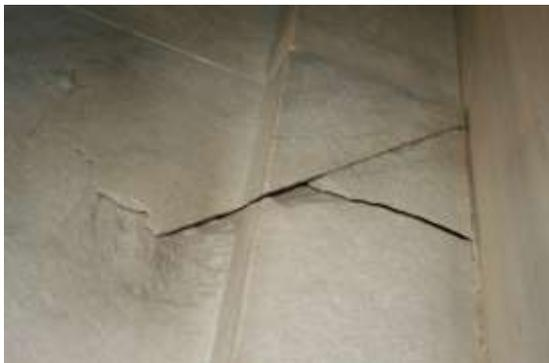
Figure 3: Corrosion based marble crack (Güneş, 2011).
