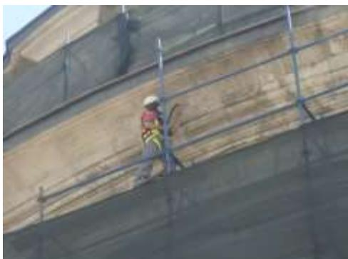
Figure 5: Sandblasting of facade (Güneş, 2011).
