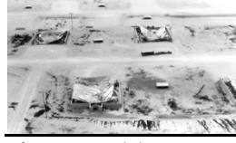
Figure (5) Accident because of Earth quake [3] Hangars at Clark Air Base destroyed by ashfall from Pinatubo eruption. Photo by E.J. Wolfe.
